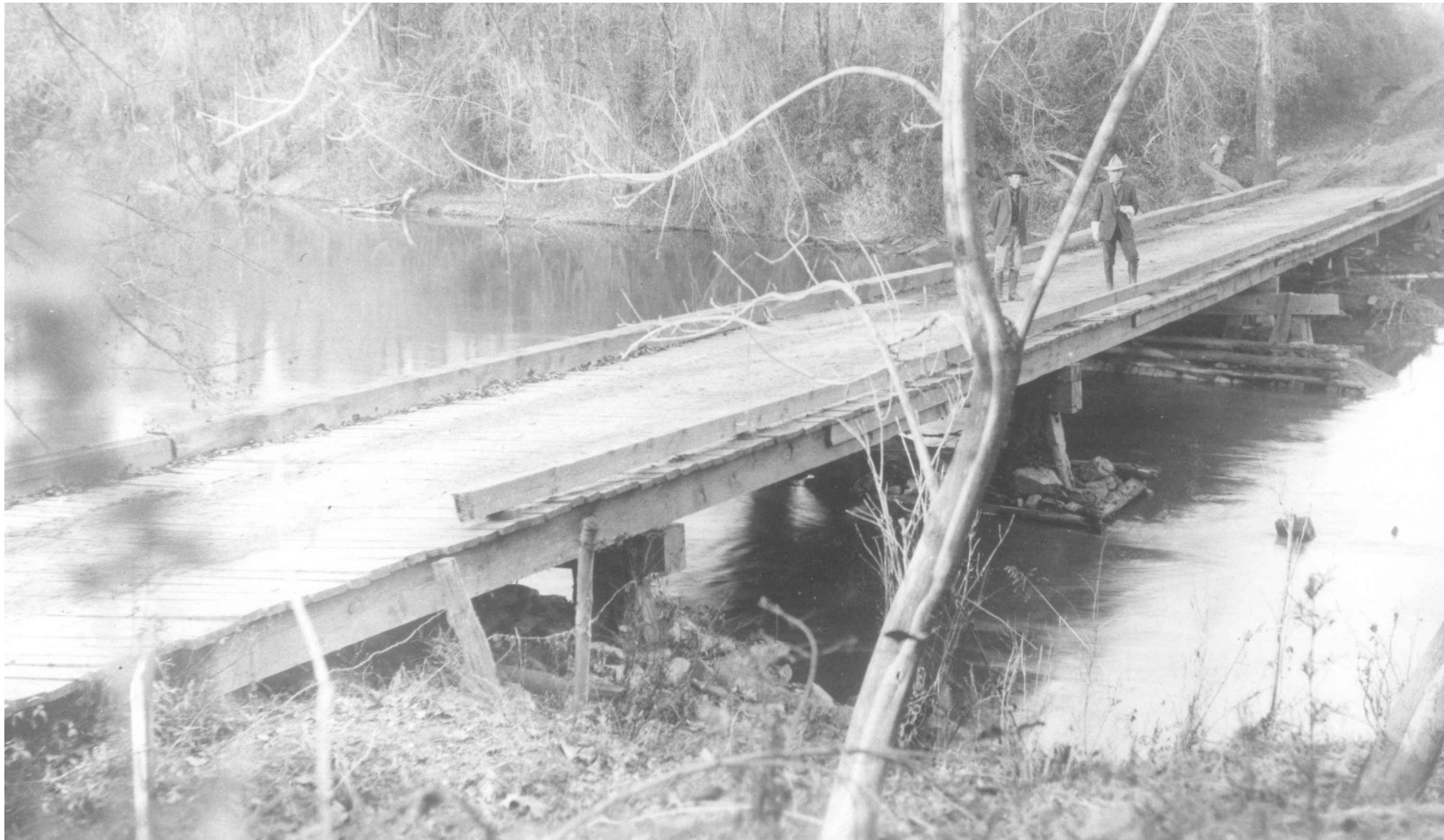
Figure 11. Constructed Assumed Downstream Construction Bridge
