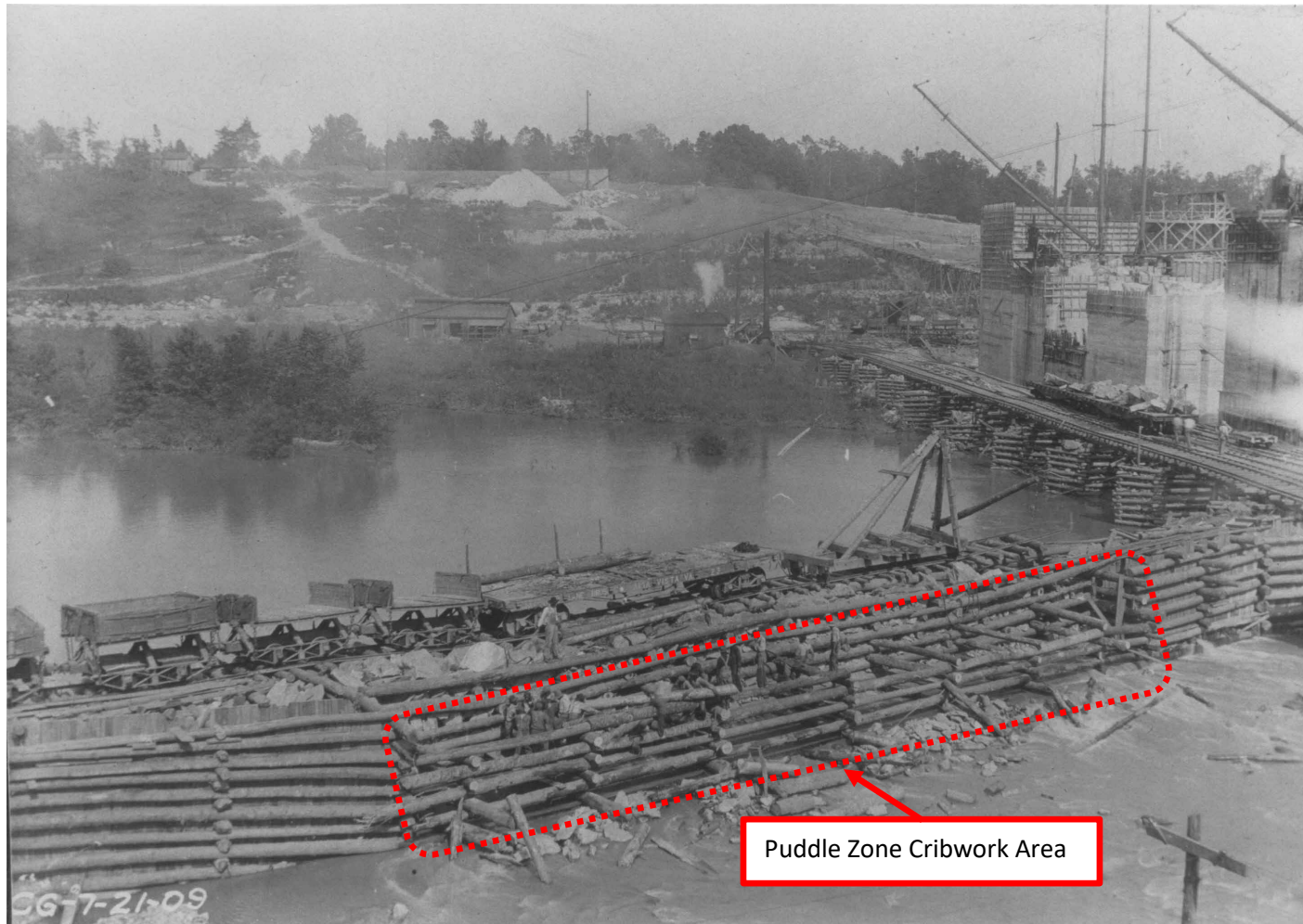
Figure 68. Upstream Second Cofferdam Puddle Zone Construction
