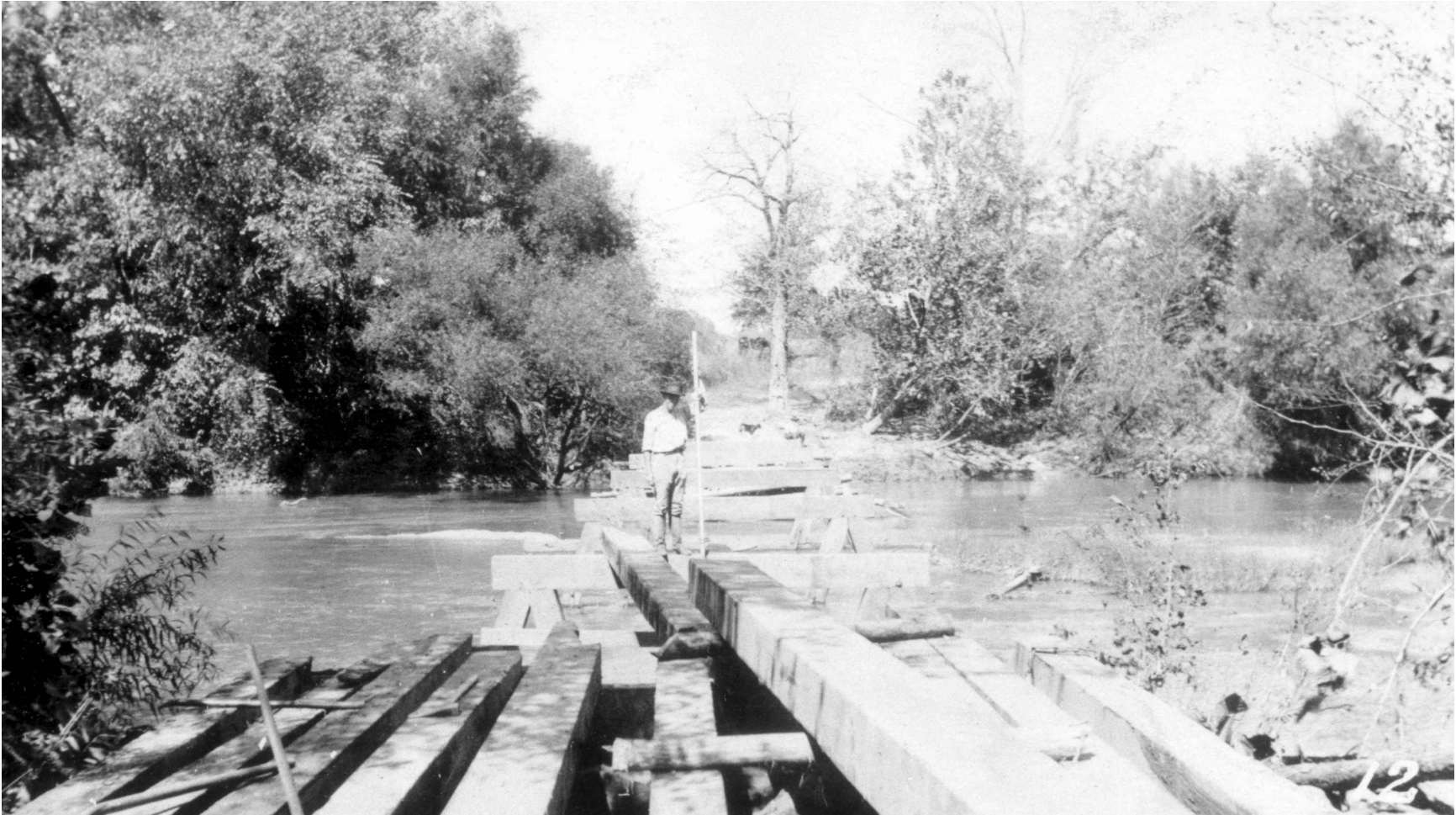
Figure 10. Construction of Assumed Downstream Construction Bridge
