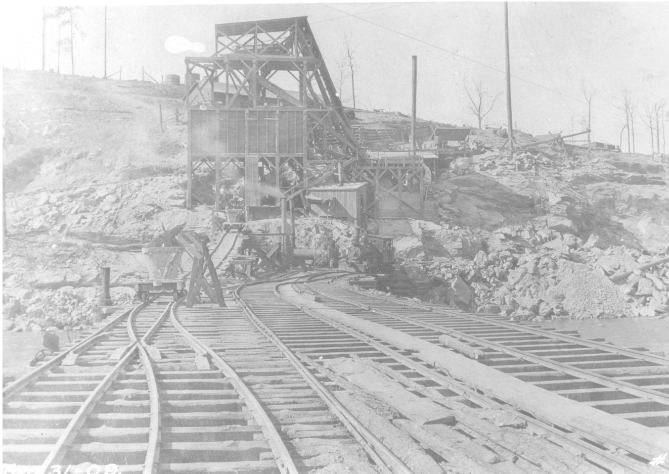
Figure 27. Completed West Batch Plant
