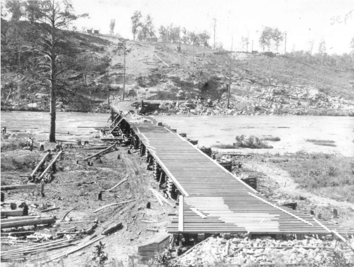
Figure 17. Filling Downstream Rock Filled Timber Crib Cofferdam Section
