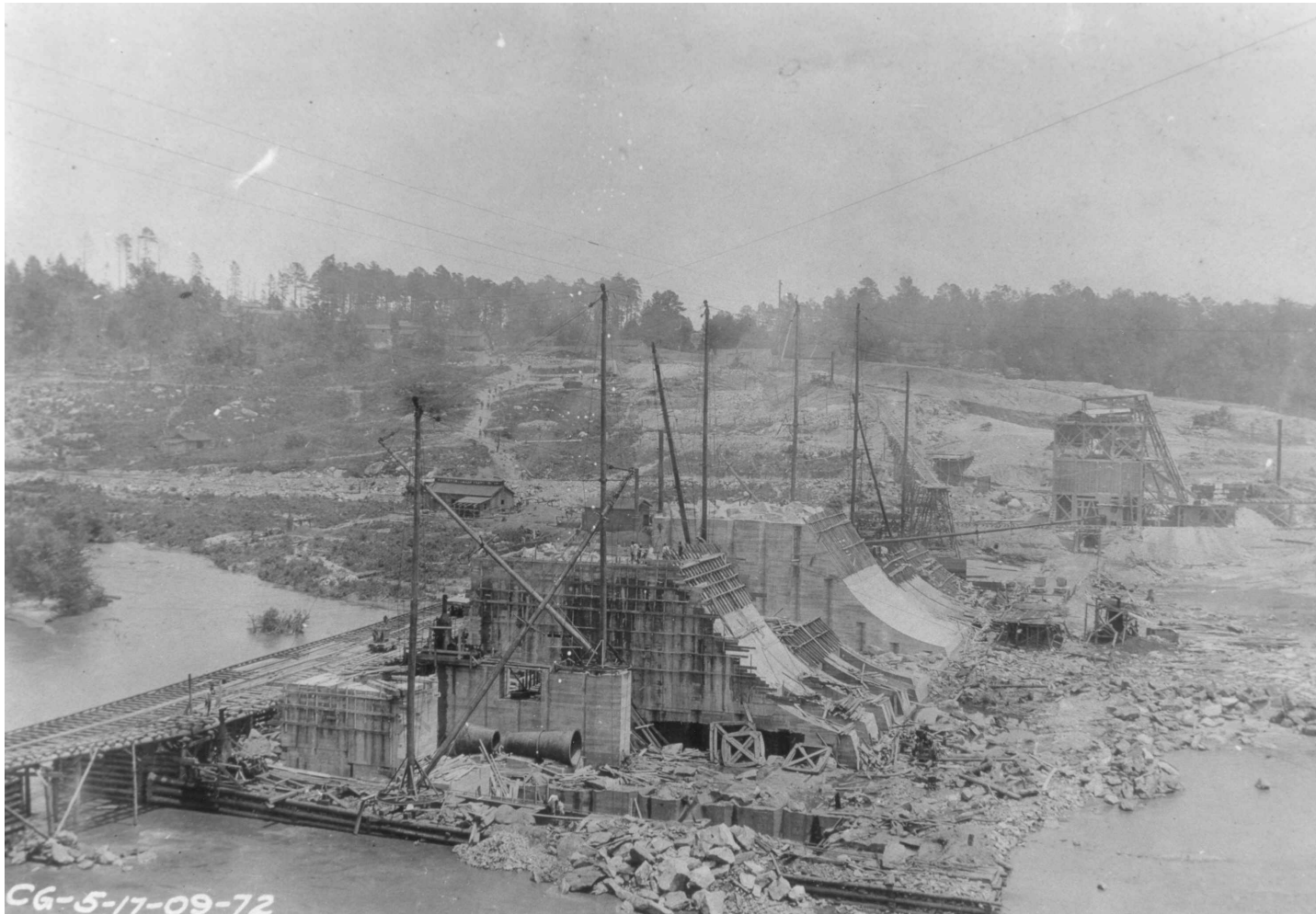
Figure 50. Westernmost Permanent Sluiceway Venturi Members
