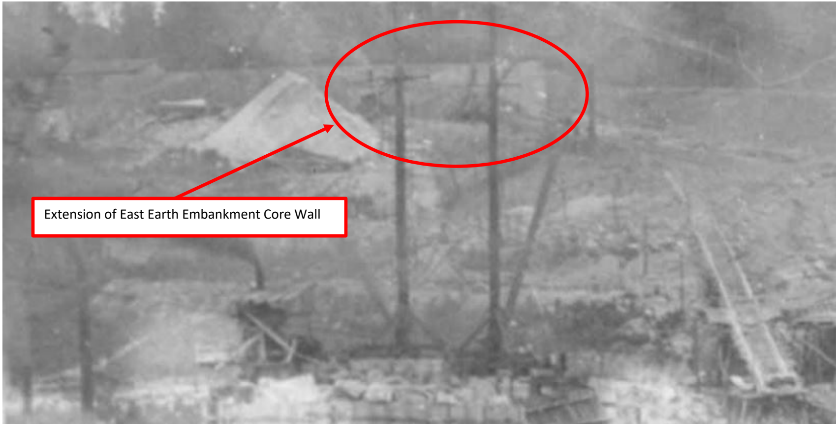
Figure 59. East Earth Embankment Core Wall as of 6/21/1909
