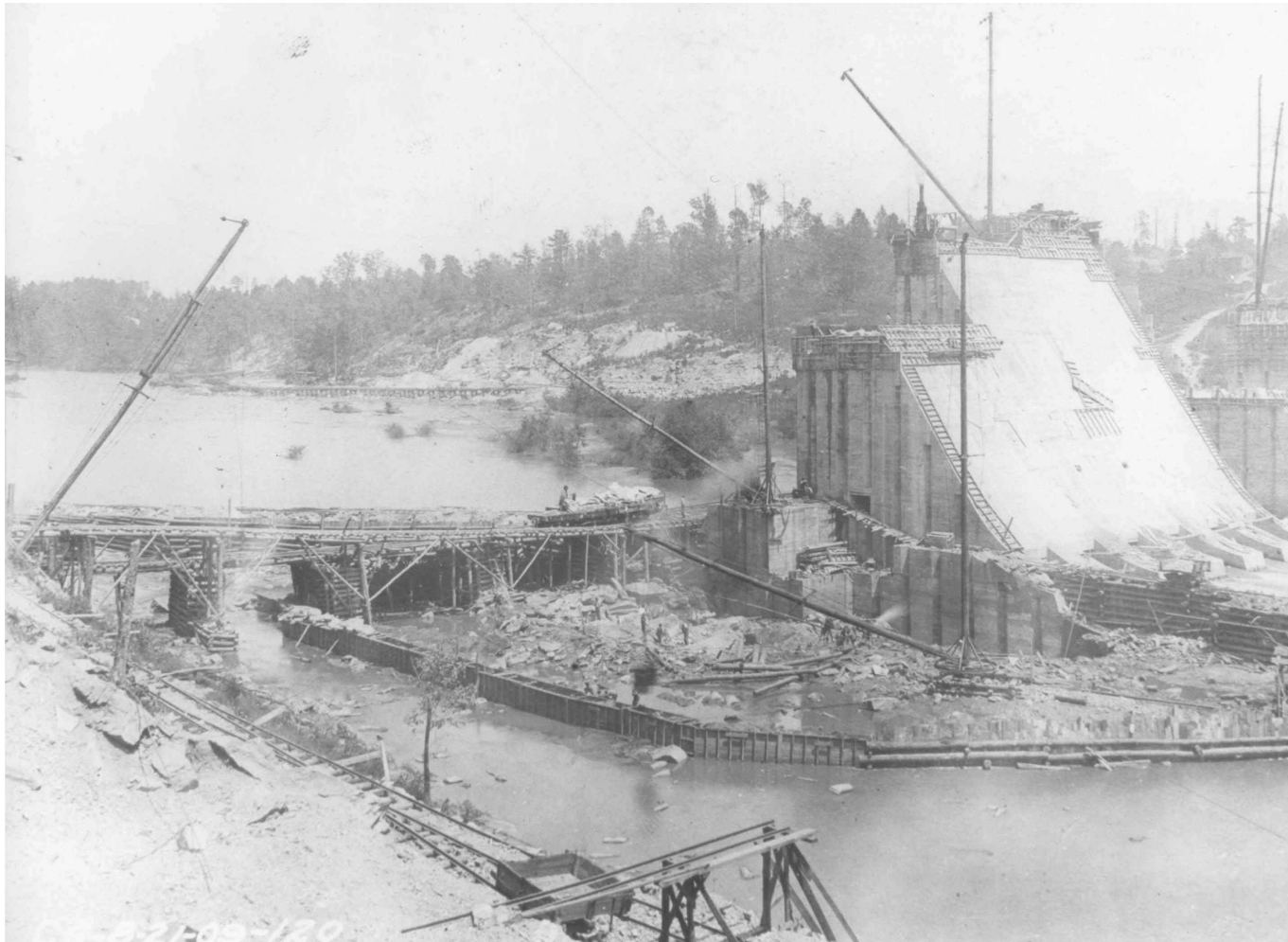
Figure 74. Powerhouse Foundation Excavation
