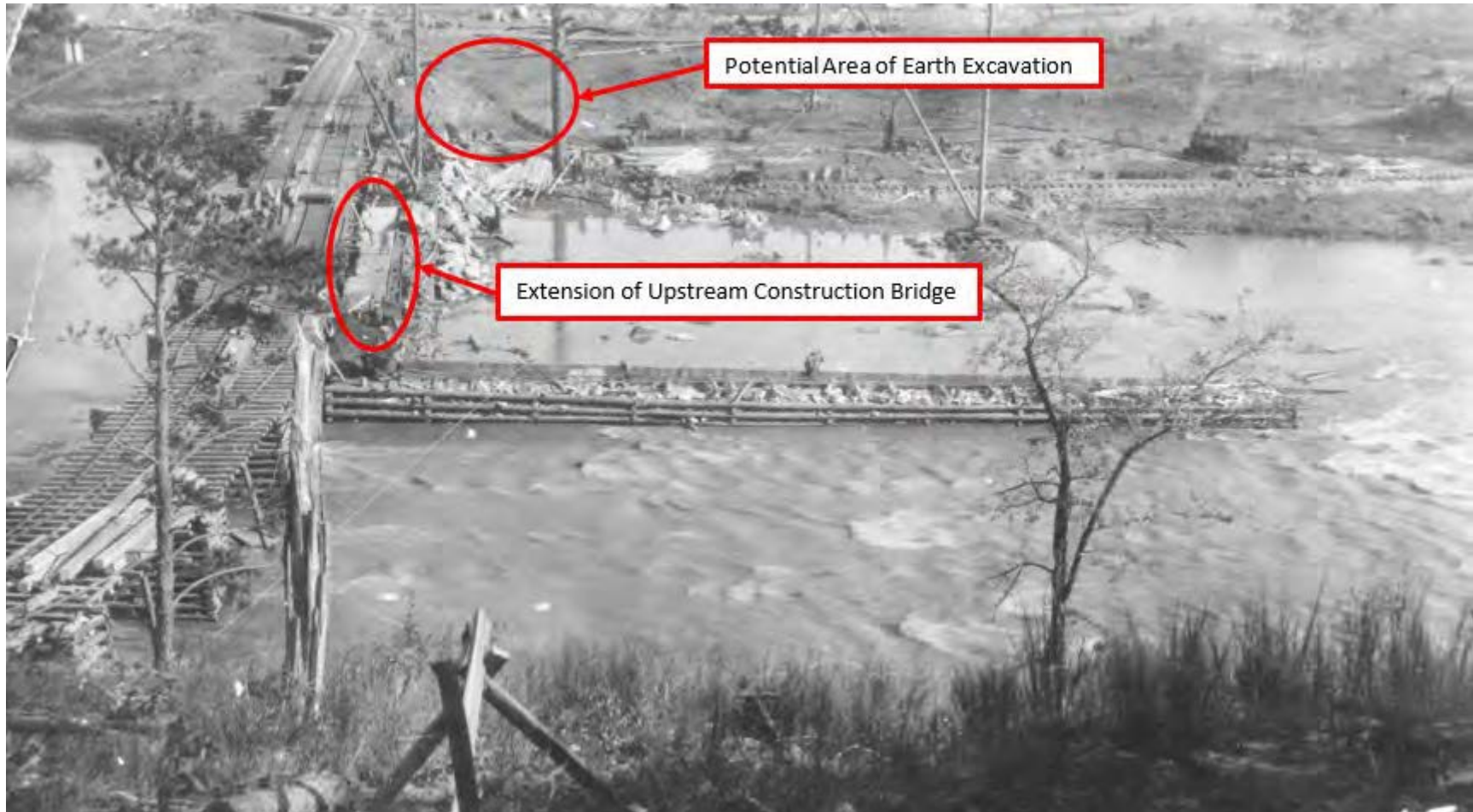
Figure 25. Apparent Extension of Upstream Construction Bridge and Potential Start of Earth Excavation
