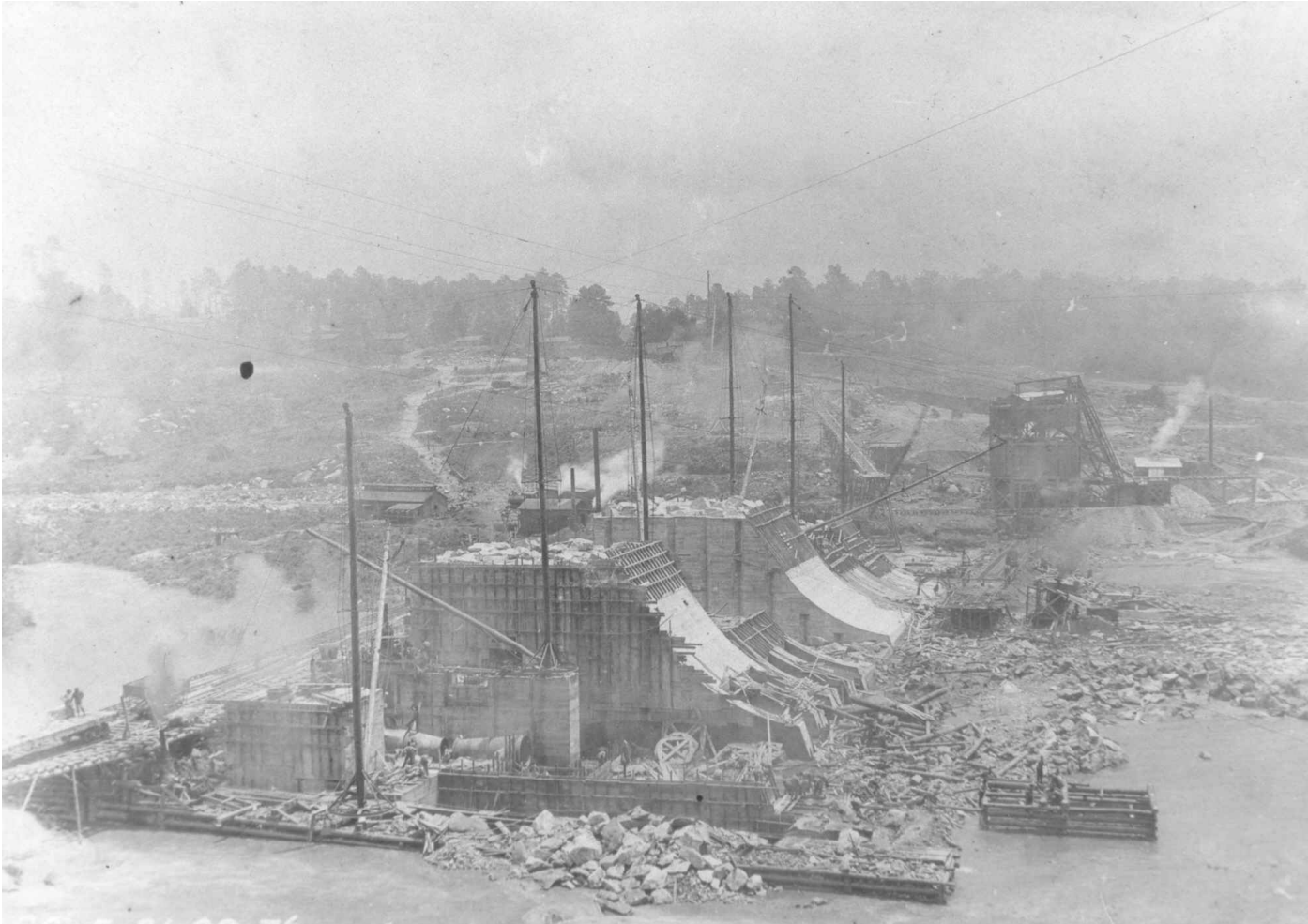
Figure 52. Form Work Extension and Crib Work Erection
