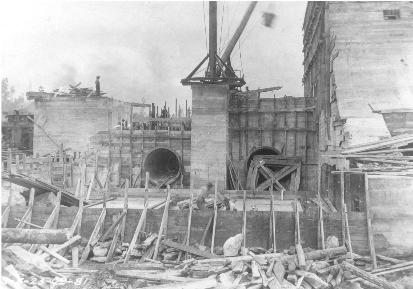
Figure 57. Concreting Westernmost Permanent Sluiceway Section on 5/25/1909
