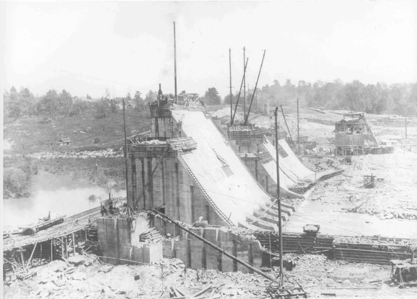
Figure 75. Construction Progress as of 8/21/1909
