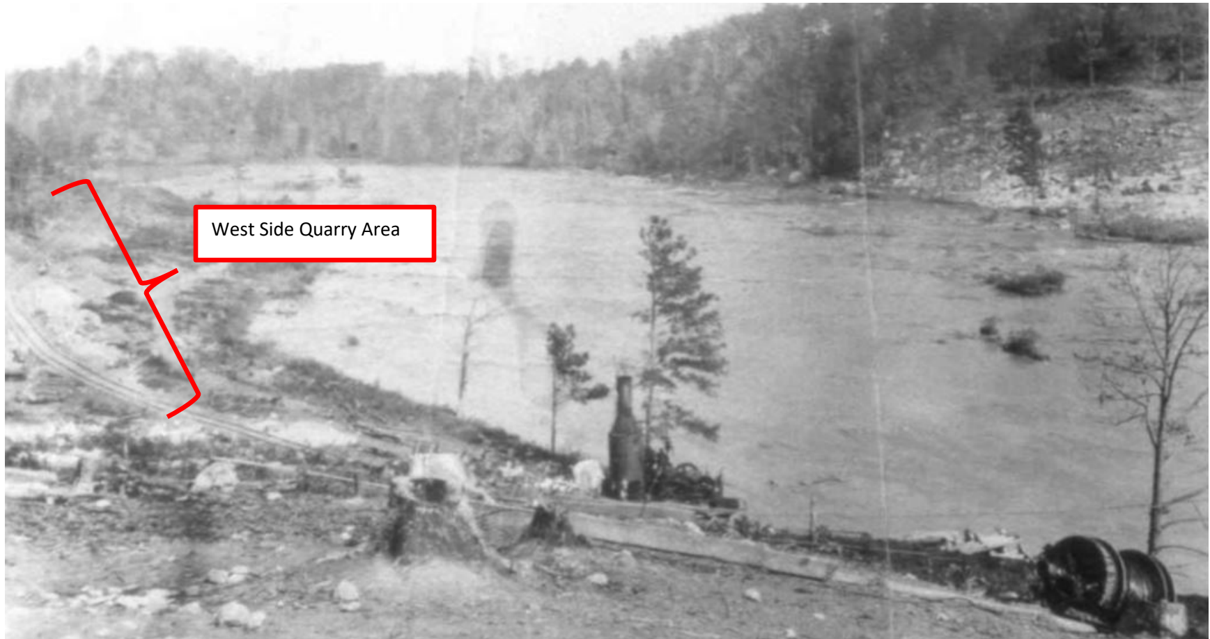
Figure 31. West Quarry Site
