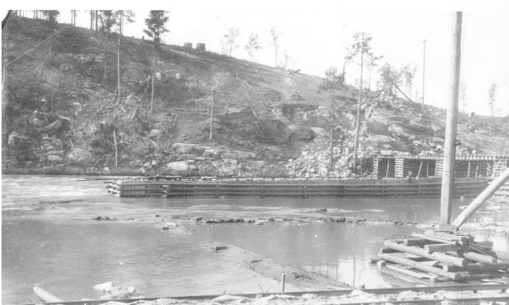
Figure 21. First Cofferdam Completed North-South Leg
