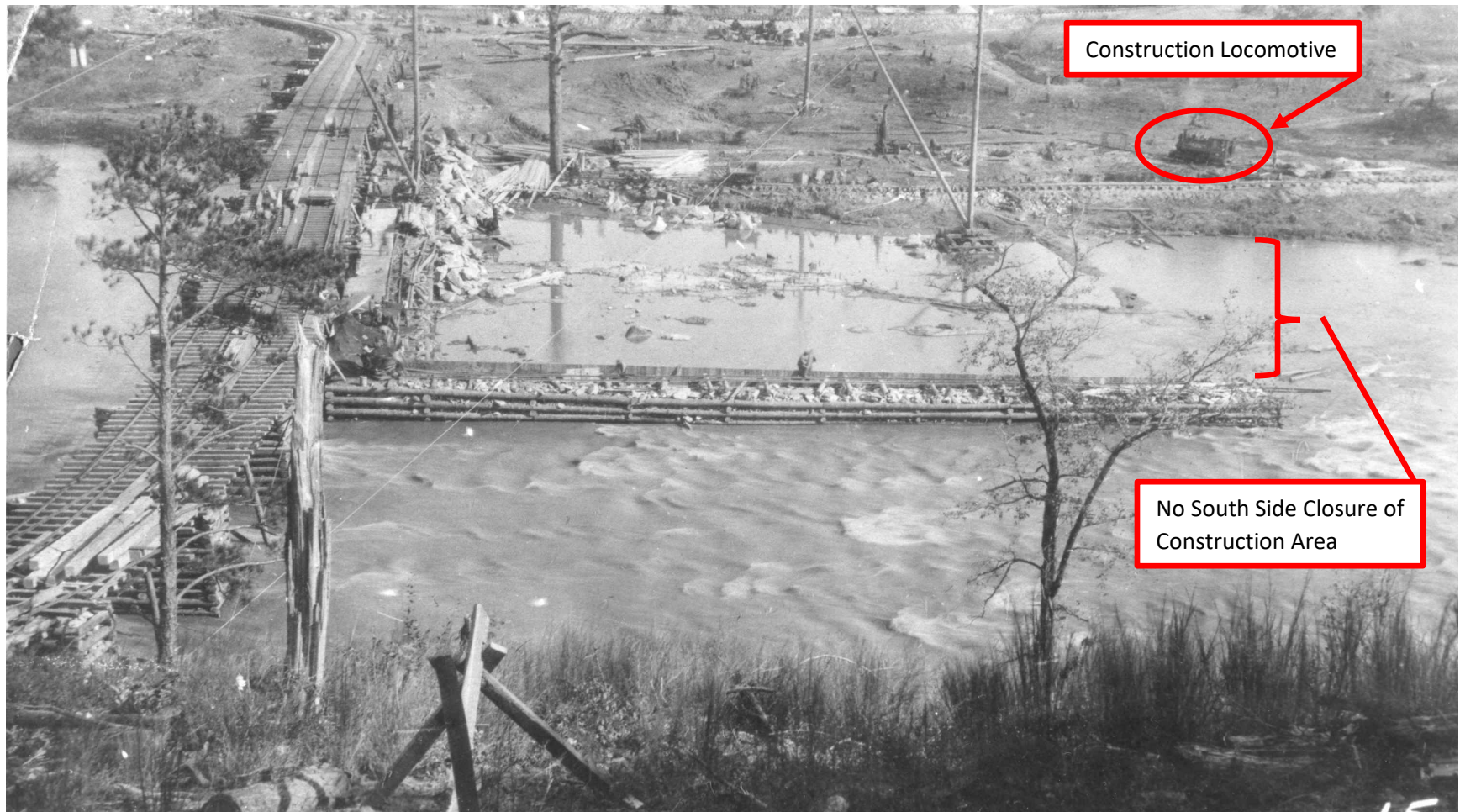
Figure 23. Partial First Cofferdam and Construction Locomotive
