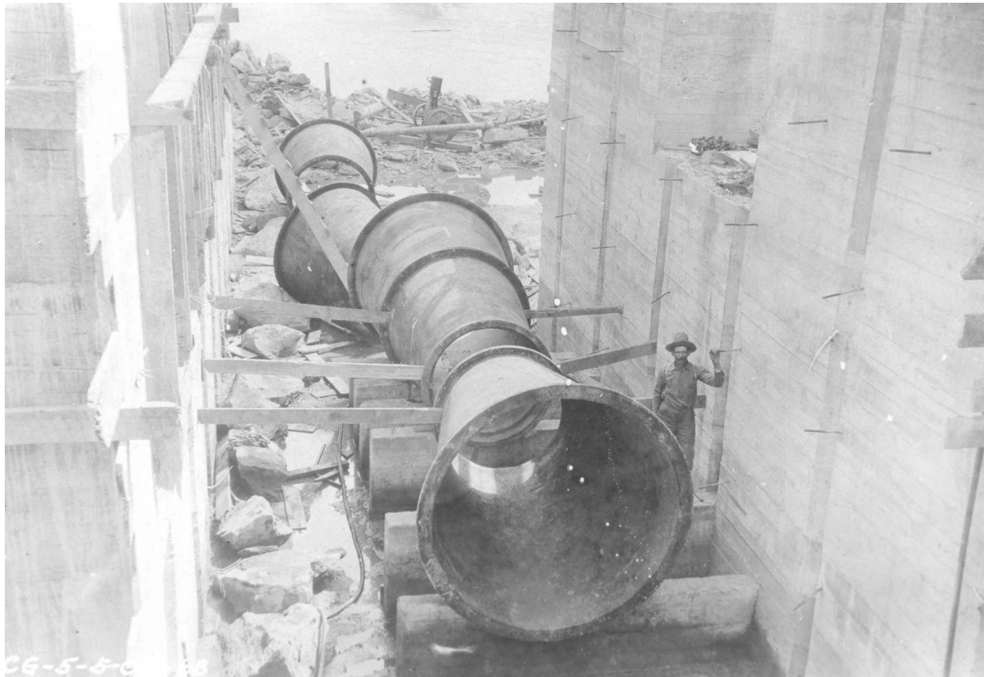
Figure 46. Easternmost Permanent Sluiceway Cast Iron Members
