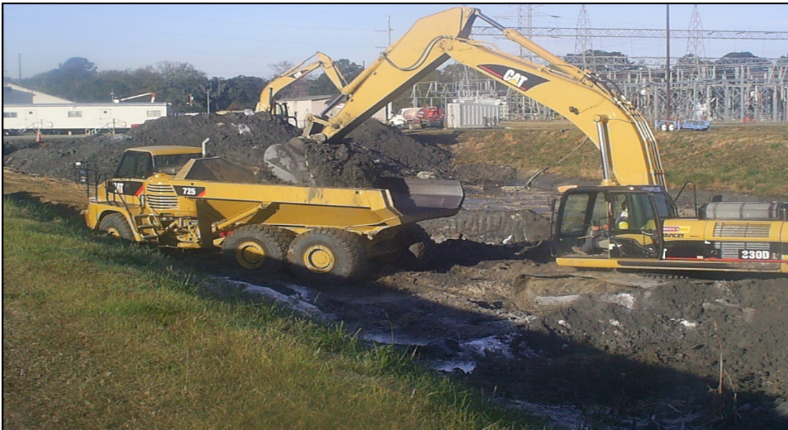
Using off-road truck to move BCWB sediment to load out area
