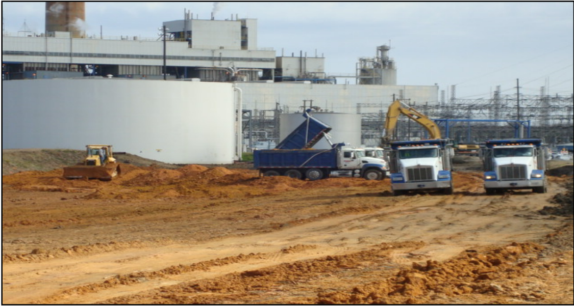
Backfilling and grading of former BCWB
