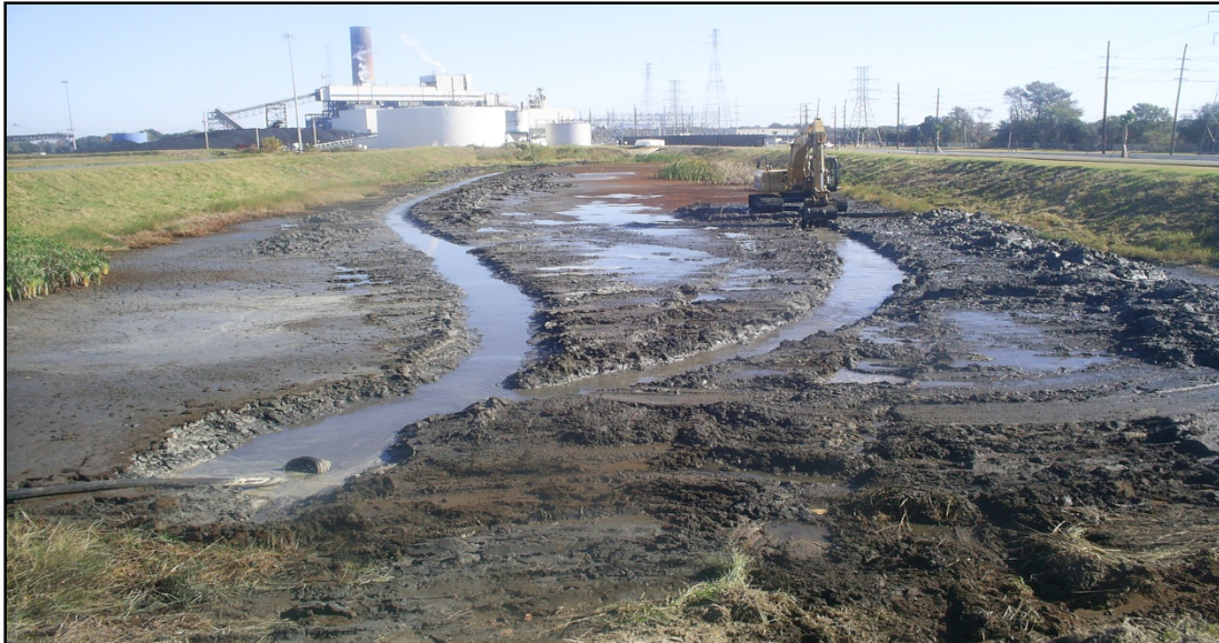
Dewatering the BCWB – Channeling water to central sump
