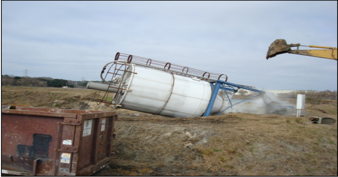
Lime silo demolition
