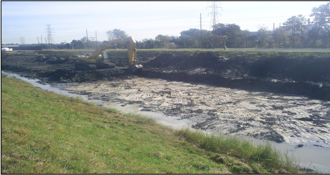
BCWB sediment was stacked up for gravity dewatering – note clay bottom on west end
