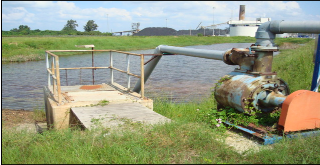
Pre-construction view to the East of the BCWB looking past the recirculation pump
