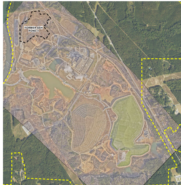
Plant Yates and the site
